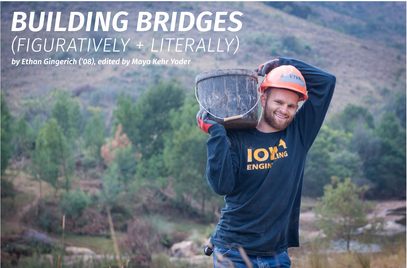
Ethan carrying concrete at Edlangeni, eSwatini Photo provided
